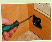
The socket was next inserted into the hole in the panel and held in position with a pair of short self-tapping screws after first drilling small pilot holes to prevent splitting.
