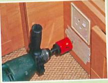
We used a Würth hole-cutter in the electric drill to make a hole in the cabinet large enough to clear the protrusions on the back of the socket.
