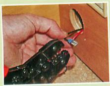
The socket ends of the cables are spade connectors and these were supplied with the kit by CAK. They were attached to the stripped cable ends with a crimping tool.
