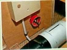
As the hole-cutter broke through on the inside of the cabinet, you could see why we'd measured, marked out and worked out for sure where to drill before starting!
