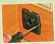
Next, the inner plinth (see pic 1, item c) was placed in position on the socket and screwed down with similar-sized screws. Their heads must recess into the plinth mouldings.
