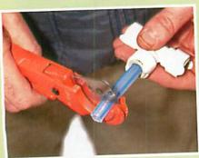
For caravans, 12mm pipe is the optimum size. You could cut the pipe with a sharp craft knife, pushing down on a cutting board, but a square cut would be difficult.
