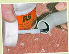
You need to brush a continuous layer around the outside of the pipe and the inside of the pipe fitting. Solvent weld actually melts the surface of the plastic...
