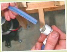
The pipe is held tight after pushing in firmly. To remove the pipe, you push the grey collar away from the pipe while also pulling on the pipe to completely remove it.
