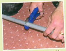
You can buy a pipe cutter suitable for all of your caravan's plastic pipes for under £10. Make sure you that you hold it square to the pipe before starting to cut.
