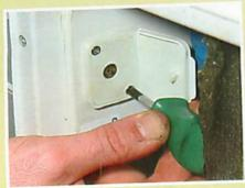
A stubby screwdriver was used in the confined space to screw in the stainless steel self-tapping screws we used. They're available quite cheaply in packs from Screwfix.
