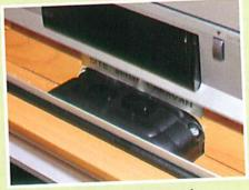
I fitted the switch, semiconcealed inside a cupboard. One button switches to the caravan aerial; the other to the external on-site TV supply. I added a label to say which is which.
