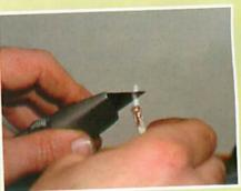
You'll need F-plugs to connect to the back of the switch. Use a very sharp knife on the coaxial cable. Cut away from your fingers or on a piece of wood or cardboard.
