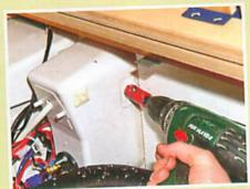
Make sure that the socket will be clear of all obstructions. It's best to drill a small pilot hole first. Then, if you've made a mistake it'll be a small one and can be corrected.
