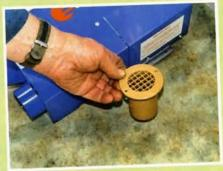
It's essential that a gas drop vent is fitted to the floor wherever a gas appliance is sited. These vents are also available from CAK Tanks, in various lengths to suit your van.
