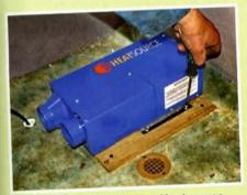
We raised the Propex Heatsource on strips of plywood to allow for the thickness of the pipe clips.
