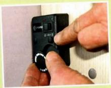
The thermostat was fitted in the living area and the wires connected. Fixing screws are concealed, with these buttons and the adjuster knob fitted last of all.
