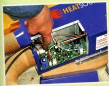
Although the 12v electrical connections need to be made by a qualified electrician, the heater-end of the cables are already fitted with plugs with matching sockets inside the unit.
