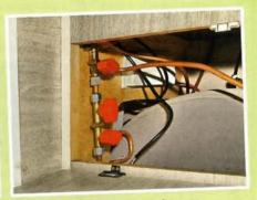
There was now an extra gas appliance to feed, so our gas fitter added an extra tap, once again supplied by CAK Tanks. It was added alongside the two existing taps in situ.
