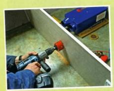
Back inside the caravan, holes were drilled into which vents could be fitted: one or two outlet vents and one for the inlet hose. A circular hole cutter does a neater job than a jigsaw.
