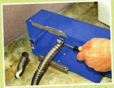
The stainless steel hoses supplied were pushed through the holes in the floor and fixed to the spigots on the base of the unit, using the hose clips that were also supplied.
