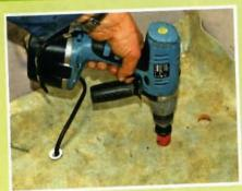
A template supplied shows you where to drill two holes for the inlet and exhaust pipes. It's essential to avoid pipes, cables and chassis rails beneath the floor.
