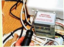
After disconnecting the mains cable and the battery terminals, the charger was unplugged and unscrewed. The 2-pin continental plug was cut off the end of the mains cable on the new charger.
