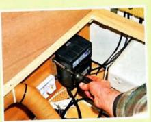
The charger's integral brackets were slotted home before refitting the cover. When screwed down, there's an air gap behind the charger and there must be clear space all round it, too.
