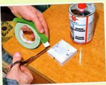
We added a switched fuse so the power could be turned off. The backplate was fitted with doublesided tape and screws after degreasing first with Würth silicone remover.
