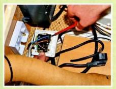
Connecting the mains cables to the switched fuse is an electrician's job. I've never understood why caravan battery chargers aren't always fitted with their very own isolator switches. At least this one is now!
