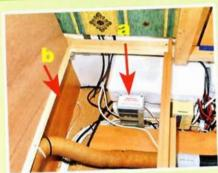
The 'old' charger (a) is almost always on or next to the battery box. I decided to fit the CAK electronic battery charger to the adjacent bulkhead panel instead.
