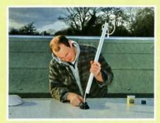
Because the aerial cable has to be inserted into the weatherproof cap, it's easier to feed the aerial wire into the mast before inserting it into the mast tube.
