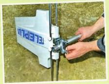
Space restrictions inside our caravan meant the mast had to be cut down, reducing the aerial height available. The aerial was fitted first before measuring and cutting the tube.
