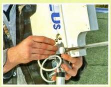
Before fitting the Teleplus aerial to the mast, remember to screw on the aerial cable. Seal it with more Vaseline to stop corrosion in future, otherwise the TV's picture quality will deteriorate over time.
