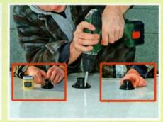
You need to seal the top flange - it swivels for sloping roofs. There's a rubber cover (right) and a spring seal (left). Smear Vaseline into the housing to lube the mast.
