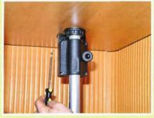
If the mast is used full-height, the clamp is best mounted on a wall. In our case, it was okay to mount the clamp on a bracket, against the roof.
