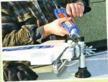
Before fitting the top cap, we used good ol' Würth Bond & Seal to make a fully waterproof seal and to ensure that the cap couldn't be blown off.
